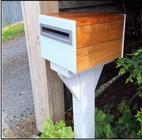
A lady brought in a letter box she had bought without realising it was intended to be incorporated into a brick wall. Roger C fixed timber panels to the top and sides and fixed it on to her old letter box post.
