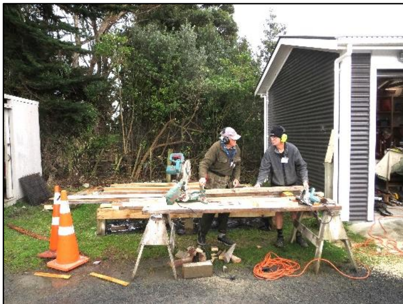
Murray C and Peter H doing the floor slab
