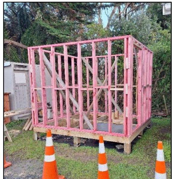
The wall framing put up in a day
