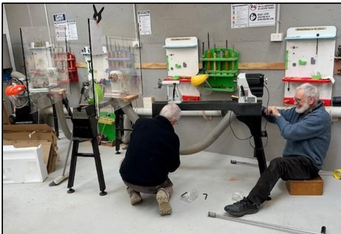
The new lathes being installed by Ian P and Marcel
