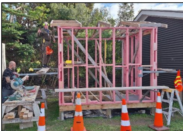
Roof trusses on with provision for a rooflights.
