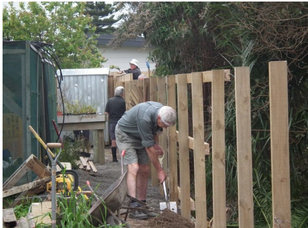
Backfilling behind the retaining board.
