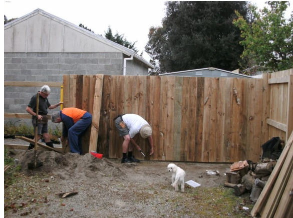
Attaching the fence palings and capping
