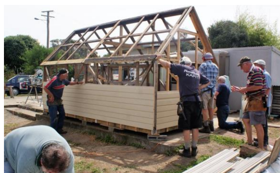
And weatherboard is being fitted.
