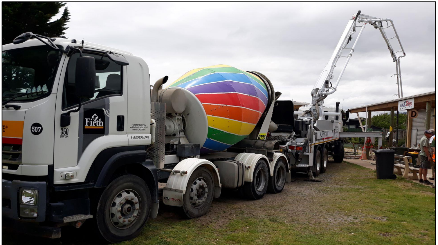
6m3 concrete pour, truck & pump with crane - just for the foundations
