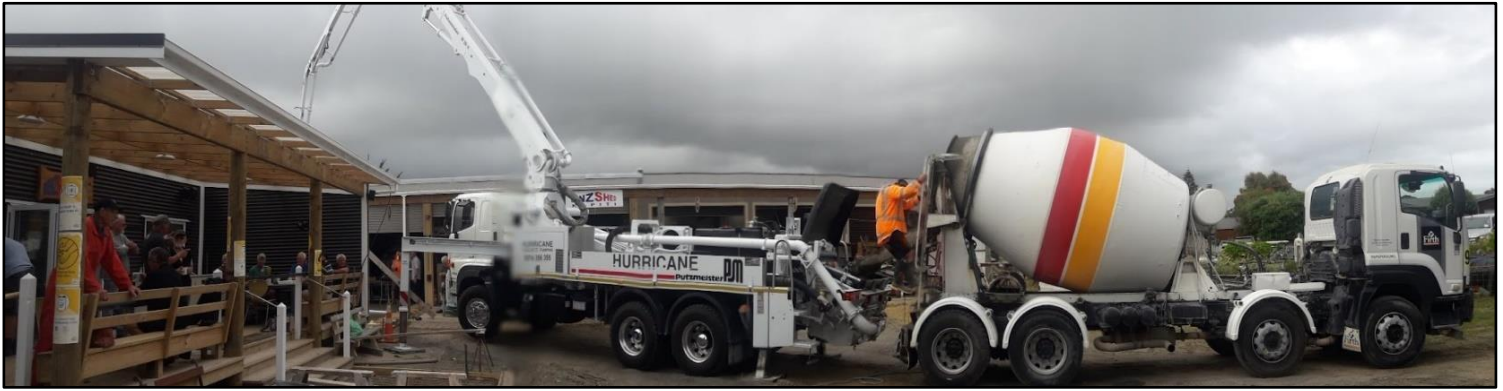
Similar setup for the foundation pour except it took 5 trucks
