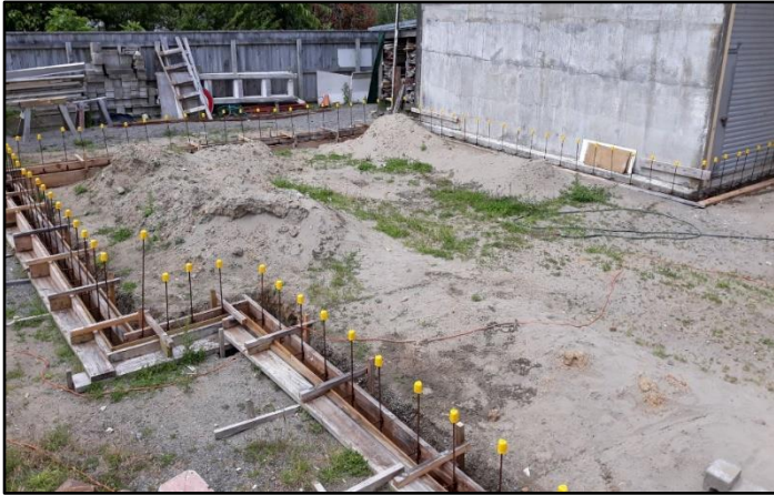
Perimeter foundations ready for the first concrete pour
