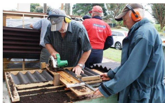
And trimming the sheets to the final size
