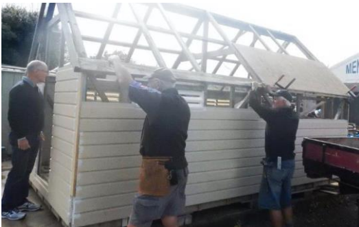
Weatherboards going on
