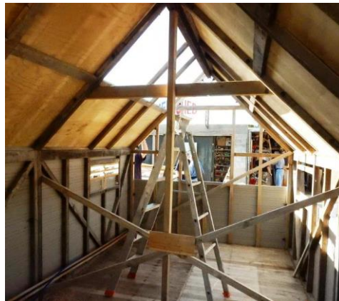
Inside the hut as the roof lining is fitted
