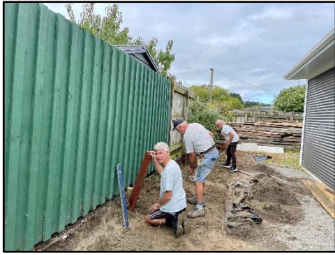
Raking and levelling the soil at the back of the workshop ready to receive four water tanks as resevoirs to take water flooding the car park and slowly release it.
