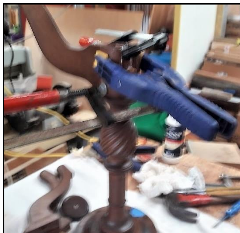
Alan W took on the job of repairing this table. Two of the feet were broken off and the centre support had to be reglued together – he did a grand job. Modern glues are so good.
