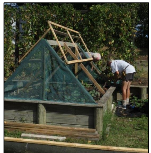
The gardeners in the process of constructing frames over the beds to support netting. They did an initial test with large mesh but the butterflies still got through so they had to go for a finer mesh
