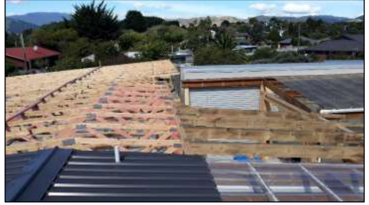
The rooftop from above now that all the roof framing is in
