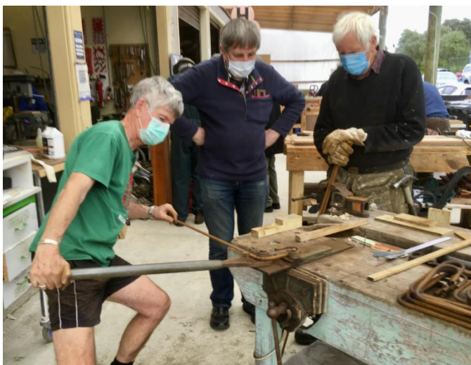
Peter H, watched by Ron Mc and Murray C, bending bars for the new workshop foundations
