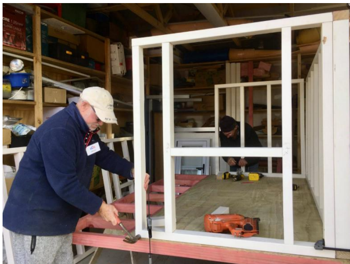
Early days of construction, putting the framing together
