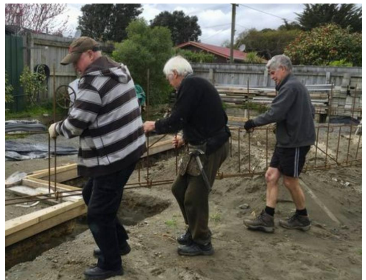
Fixing reinforcement in workshop foundations ready for concrete pour
